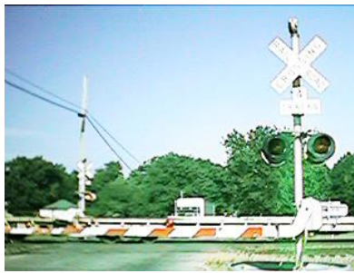
A Guarded Railroad Crossing
